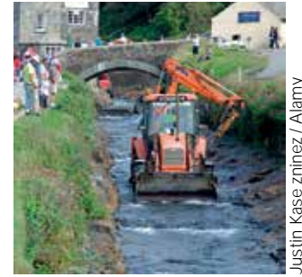
A digger deepening River Valency, Boscastle
