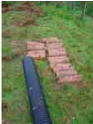
Photo 4: Tile drains removed, plastic pipe ready to be installed
